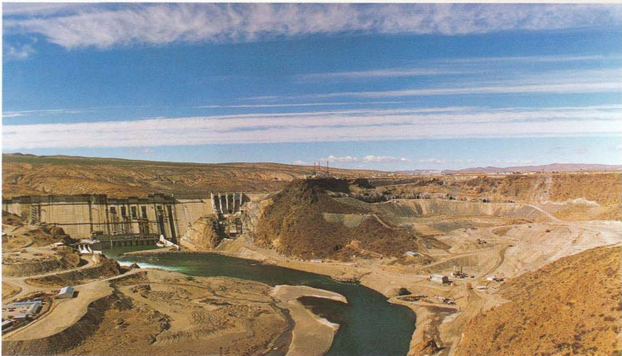
General view of the site
