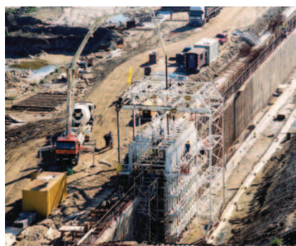
Construction of the civil works and capping beam
