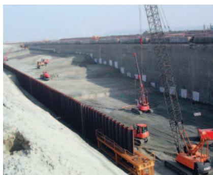
Sheet piling, anchors and backfilling behind the quay
