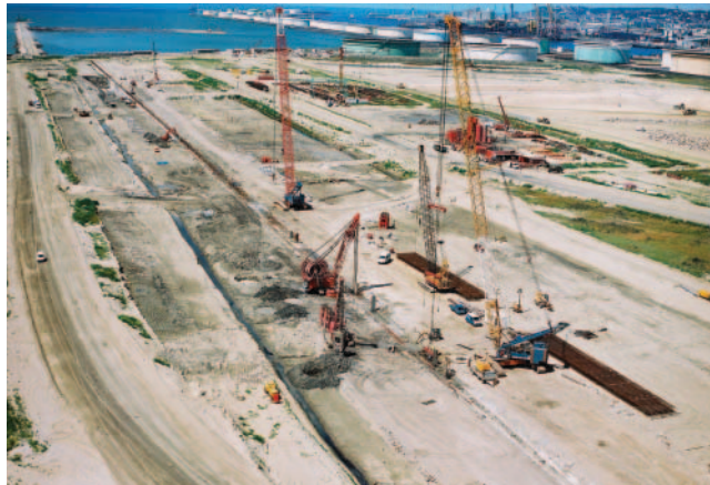
Diaphragm wall construction of the quay wall
