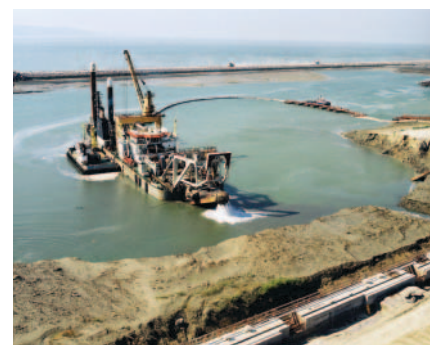
Dredging of the harbour in front of the quay wall
