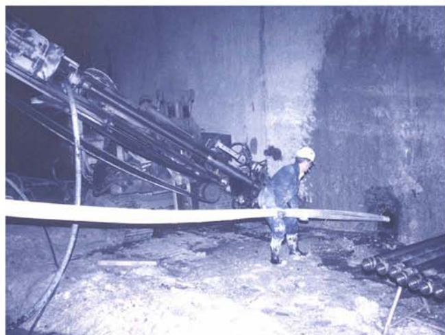
Installing a ground anchor
