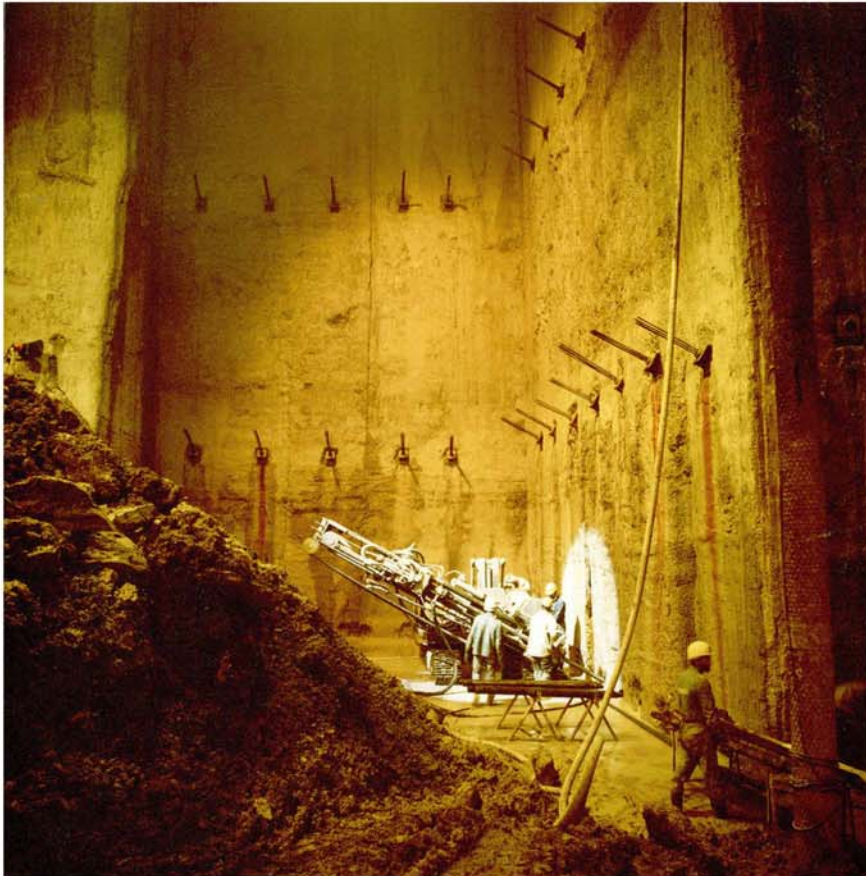
Drilling for the third row of anchor installation
