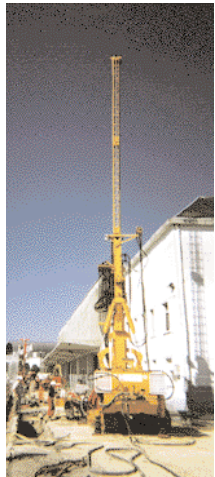
Jet grouting rig
