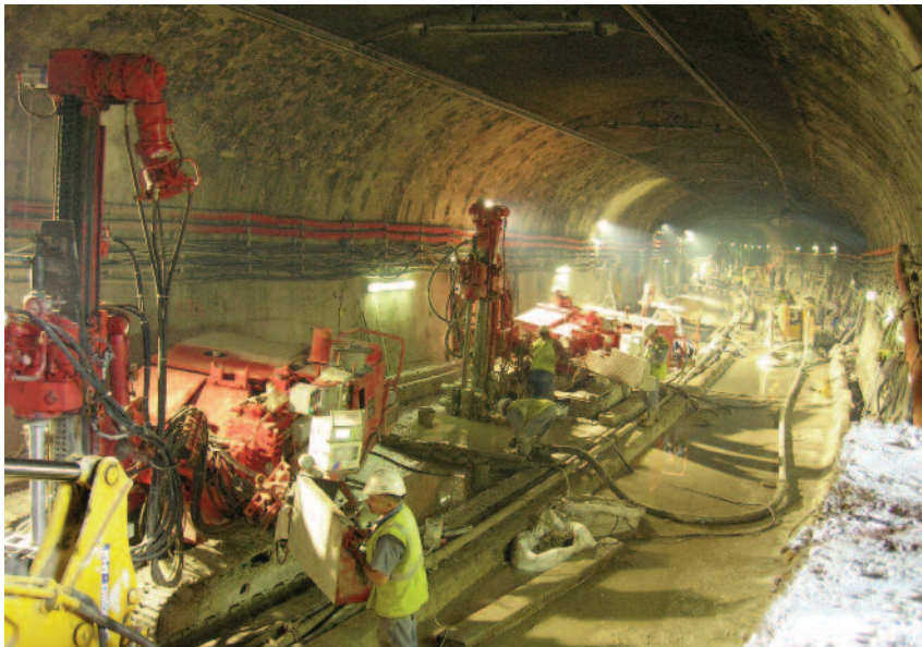
View of the tunnel with drilling rigs in action
