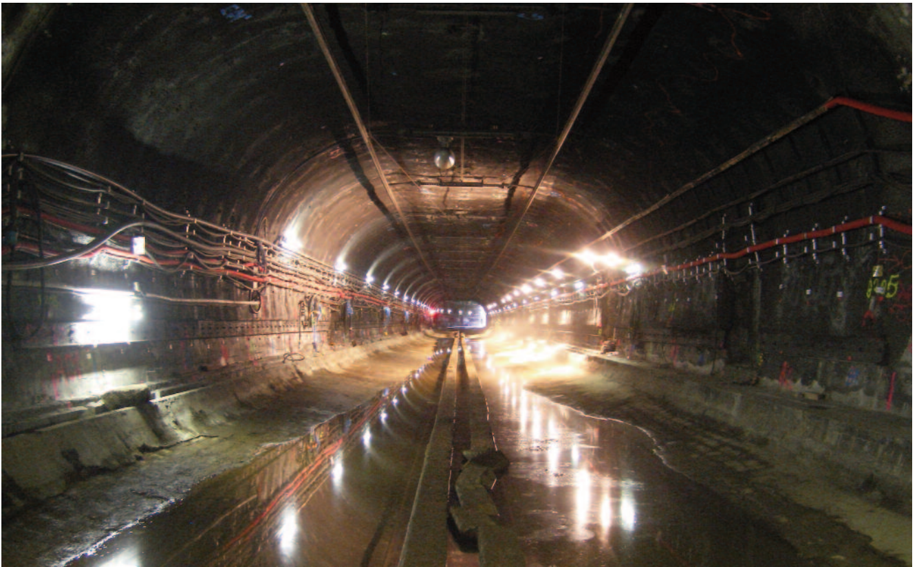
View of the tunnel after removal of the rails and ballast
