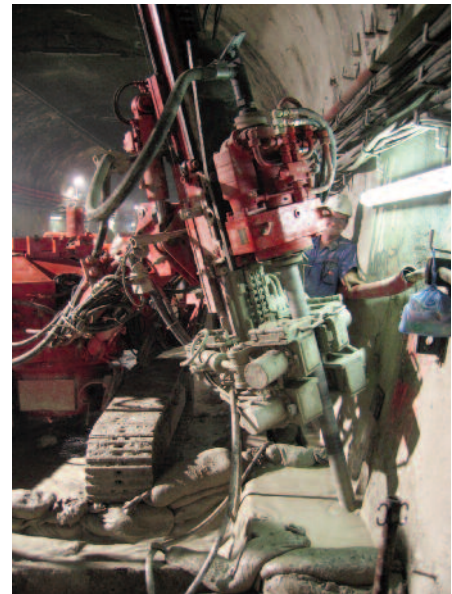
Producing a jet grouting column under the side wall
