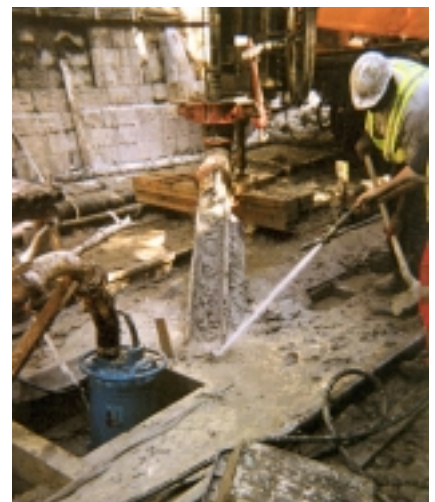
Double jet column during execution
