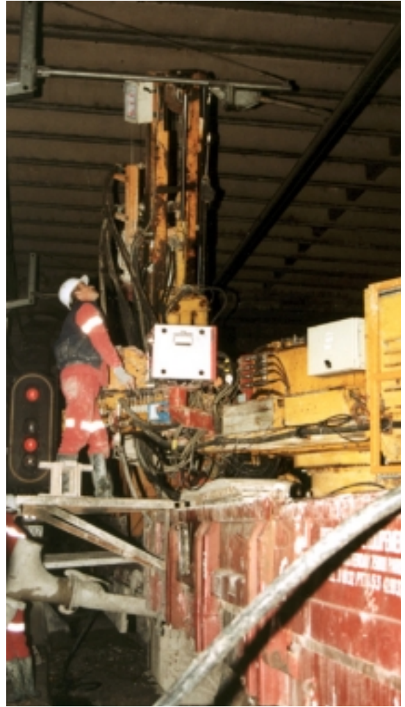
Producing columns within tunnel area from a works train
