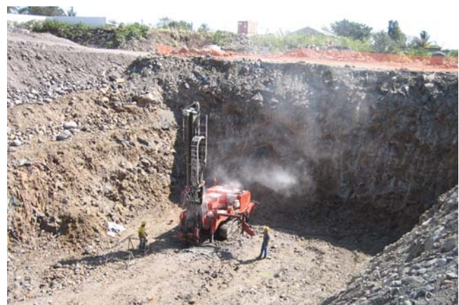
Presplitting and blasting for the P1 Pier barrettes, left bank
