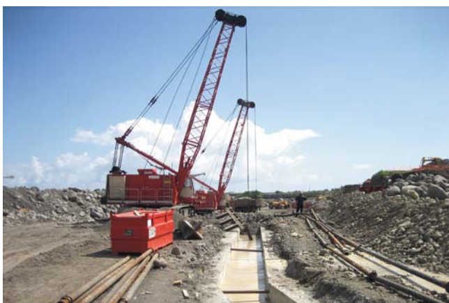
Diaphragm wall excavation, right bank
