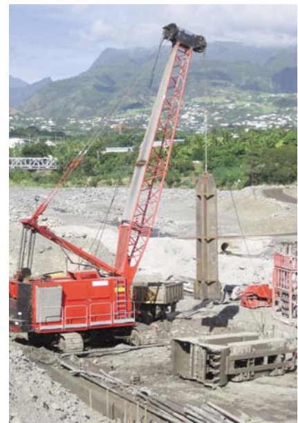
Trepanning for excavation of barrettes on the P2 pier
