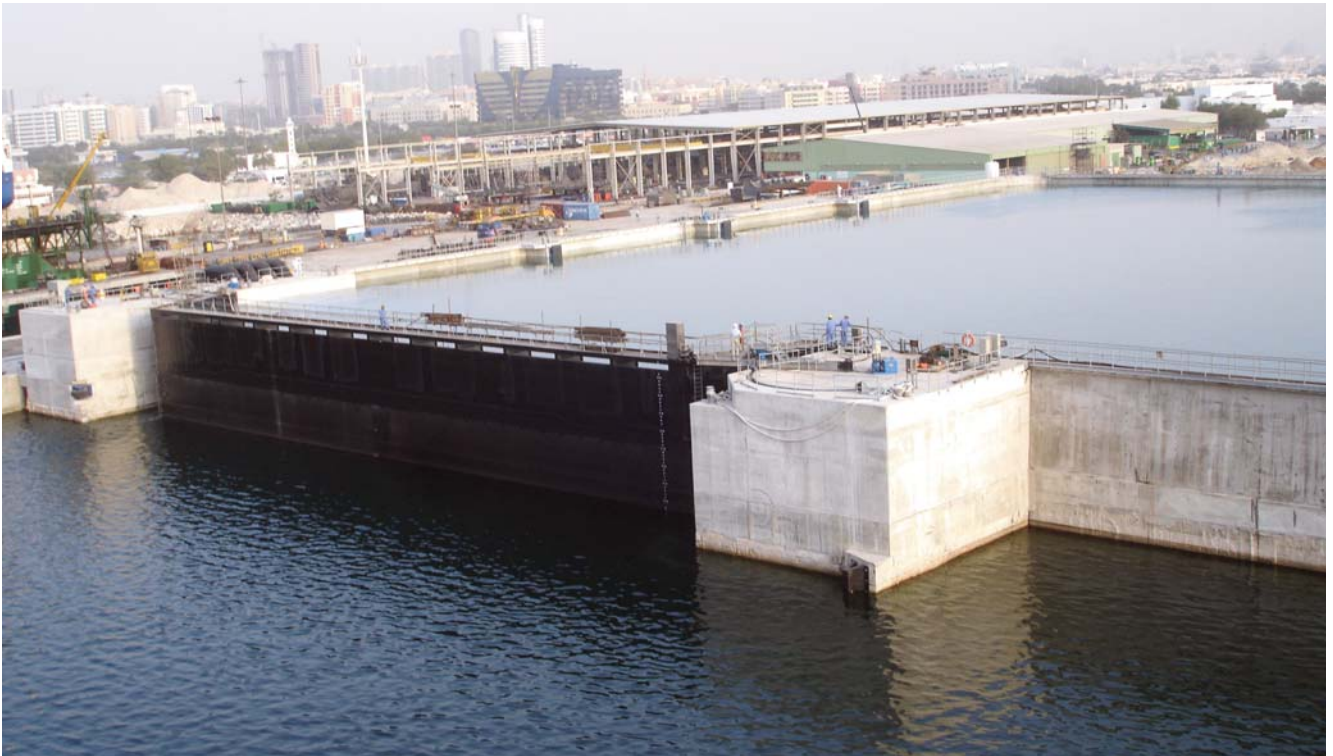
Launching facility completed
