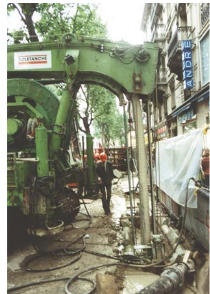
Latine Hydrofraise at work on the diaphragm wall
