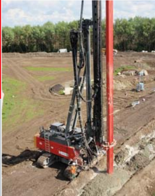
FRANCE - Lewardé 600m of Geomix® cut-off wall
