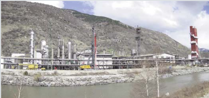
SWITZERLAND - Viège 47,000m² of Geomix® cut-off wall
