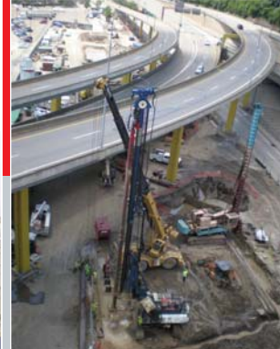
UNITED STATES - Pittsburgh North Shore Collector 10,000m² of Geomix® retaining wall
