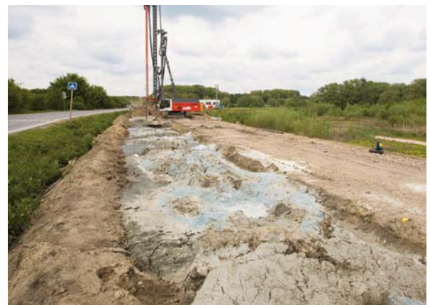
The soil/cement mix can achieve compression strengths of around 6MPa and permeability values of around 10 -6 m/s.
