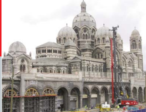
FRANCE - Marseille Axe Littoral 1,700m² of Geomix® retaining wall
