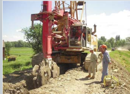
POLAND - Mielec Stary Bren embankments 2,000m² of Geomix® cut-off wall
