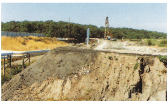
Diaphragm wall under construction from perimeter dyke
