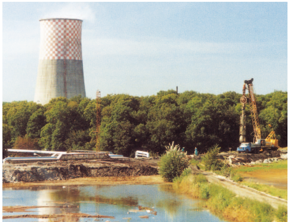
Overview of waste disposal site
