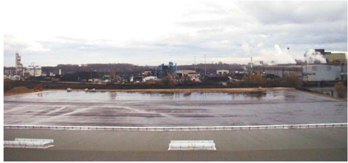
View of the completed platform
