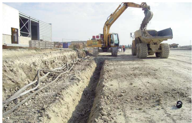
Excavating the preliminary trench
