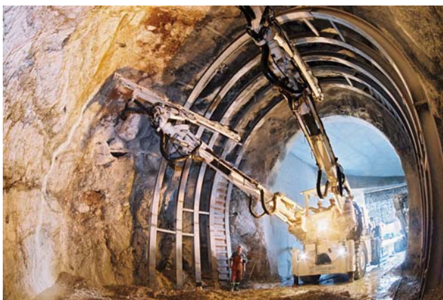
The Robofore used for drilling from the downstream tunnel
