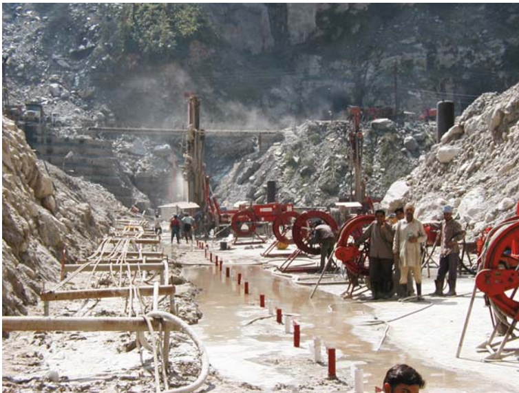
Constructing the grouted curtain
