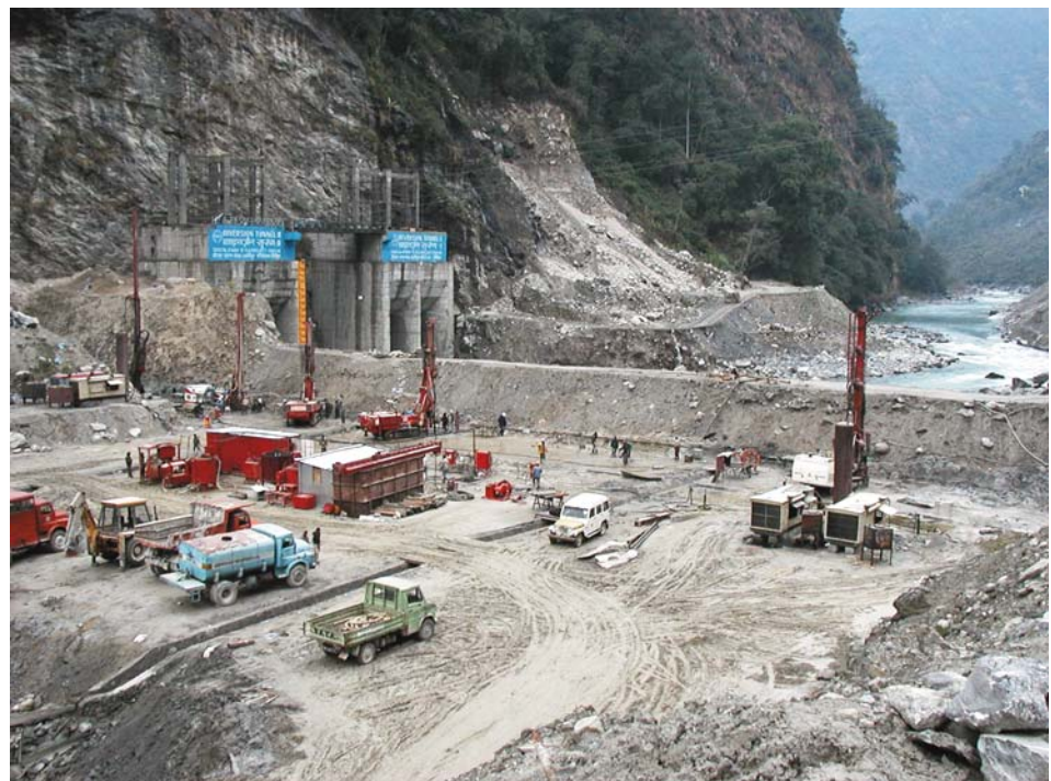
Jet grouting and grouting works on the upstream cofferdam
