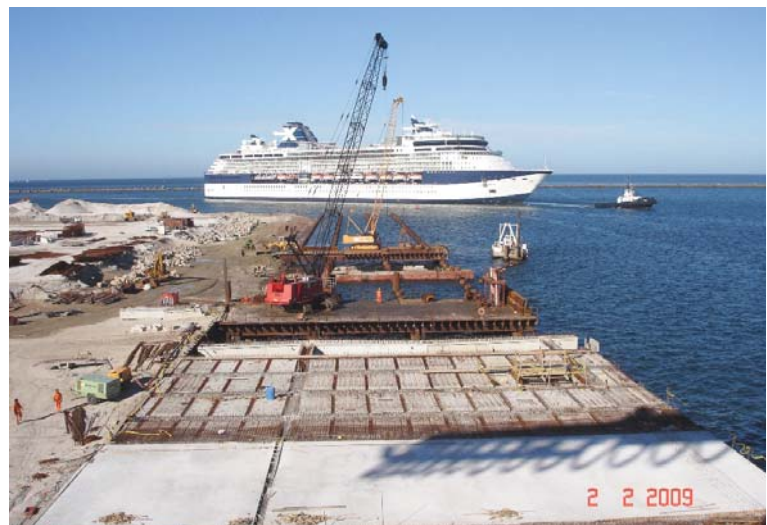
Constructing the quay's framework with prefabricated slabs and beams
