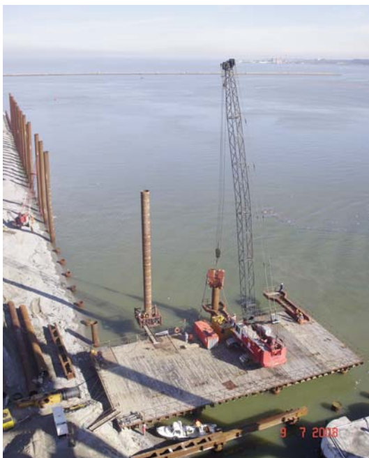
Driving in the piles from the mobile work platform using a vibrating hammer
