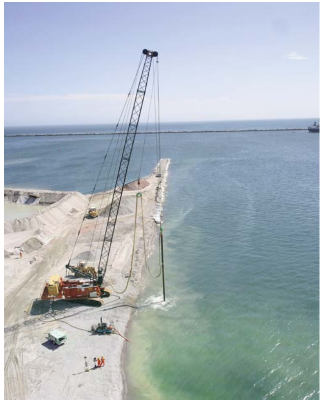
Vibroflotation in order to consolidate the reclaimed area
