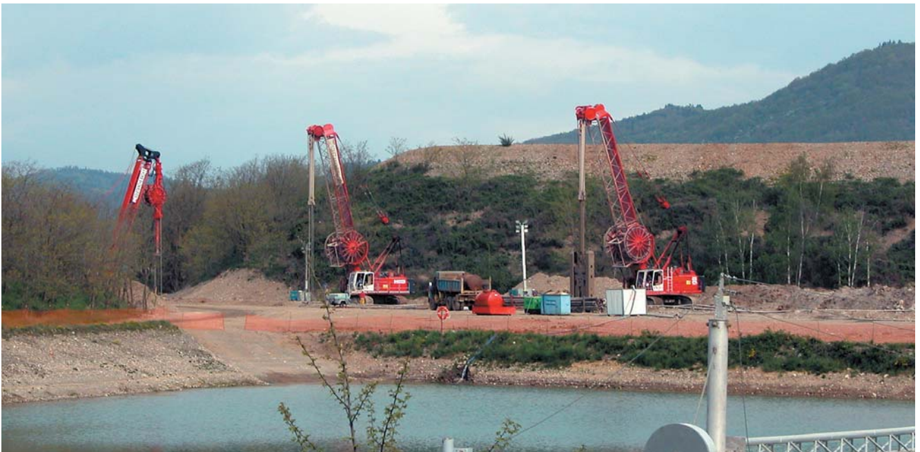
Overall picture of the jobsite
