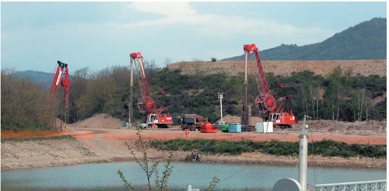
Overall picture of the jobsite
