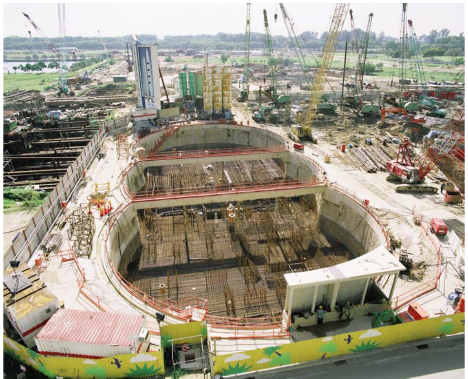
View of the excavated basement with exposed barrette heads
