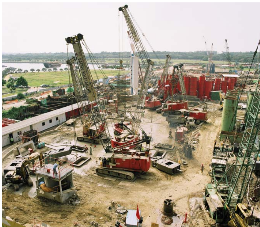
General view of construction with 5 rigs working
