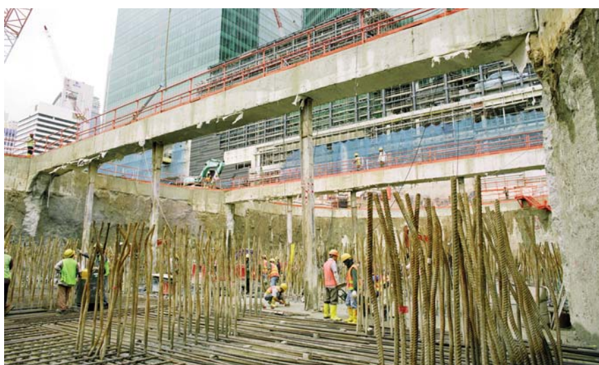
Steelfixing for the 3m thick base slab underway
