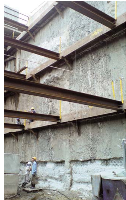
Diaphragm wall with struts on Thu Thiem side
