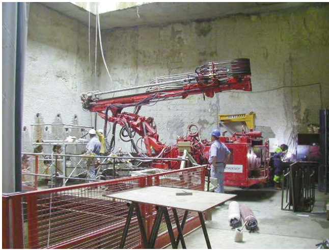
Grouting operation in the Victor Hugo shaft
