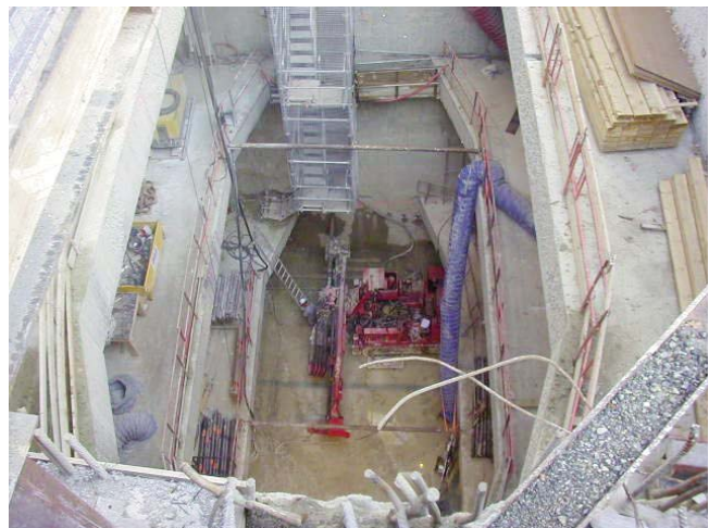
Construction of the pipe roofing
