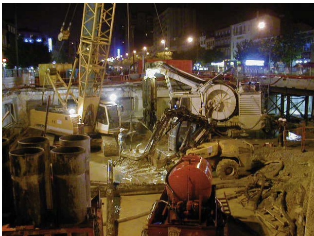
Excavation of the diaphragm wall using an HC03
