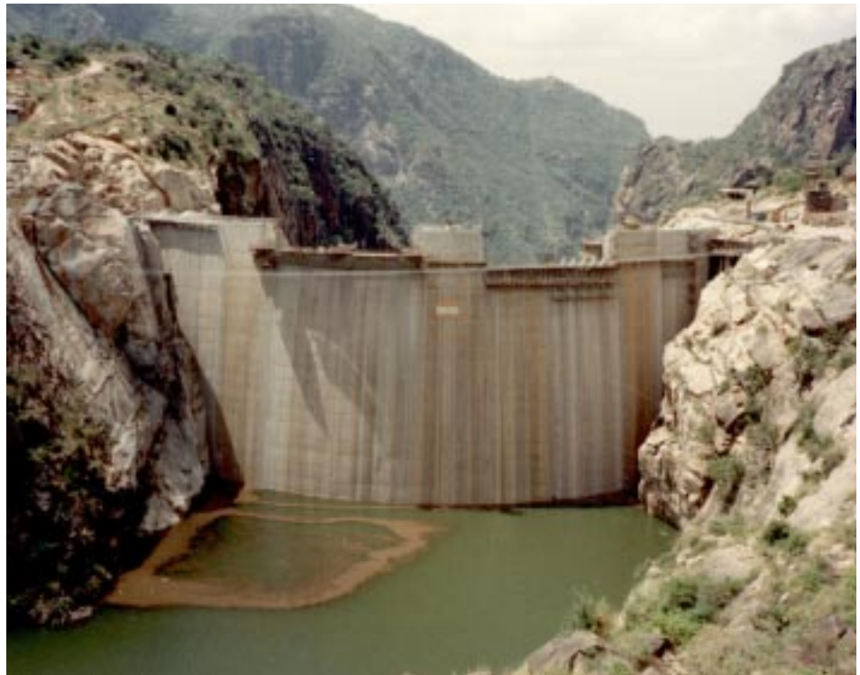
The completed dam
