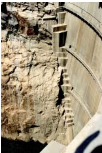
View downstream of the right abutment
