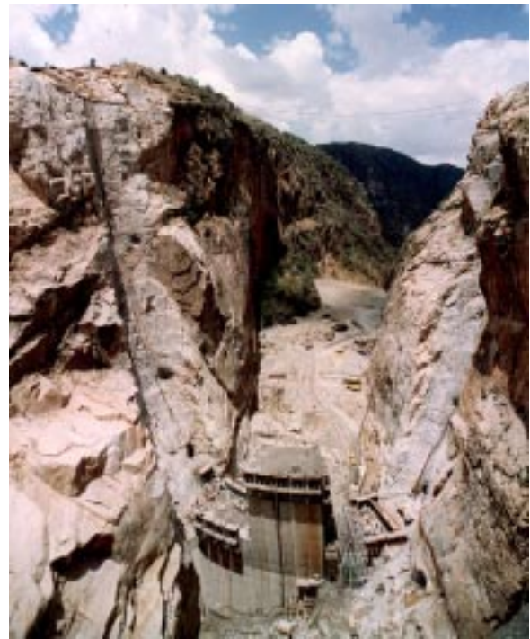
The gorge after excavation to foundation level
