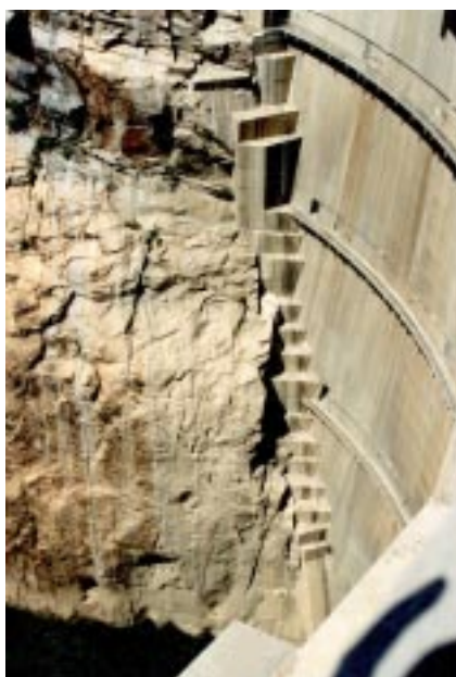
View downstream of the right abutment
