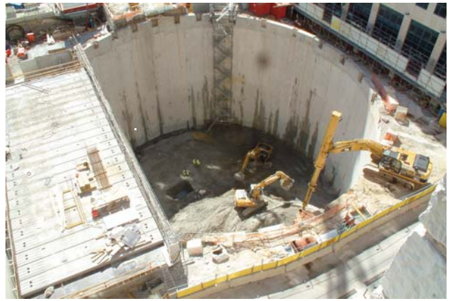
Earth moving at the final depth
