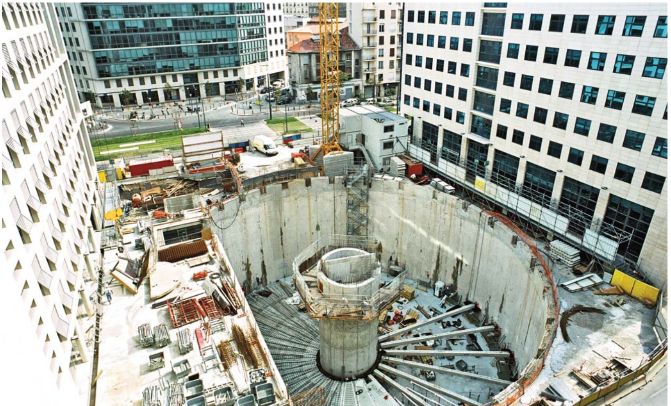
Construction of the central core and installation of the helical ceilings
