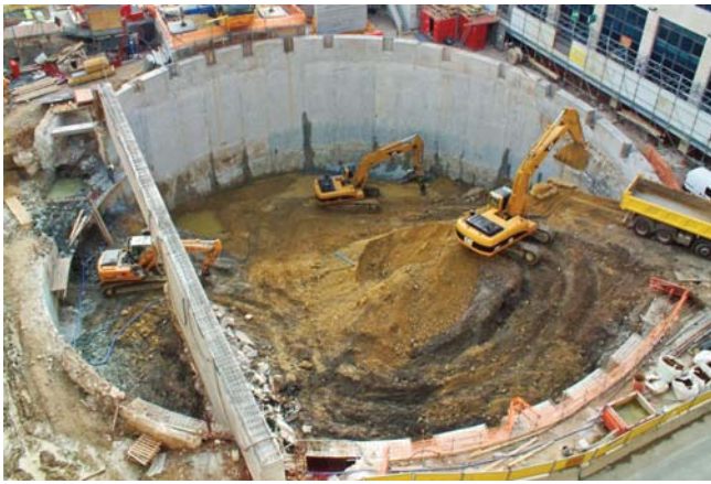
Open-cut earth moving with concomitant construction of the reception building
