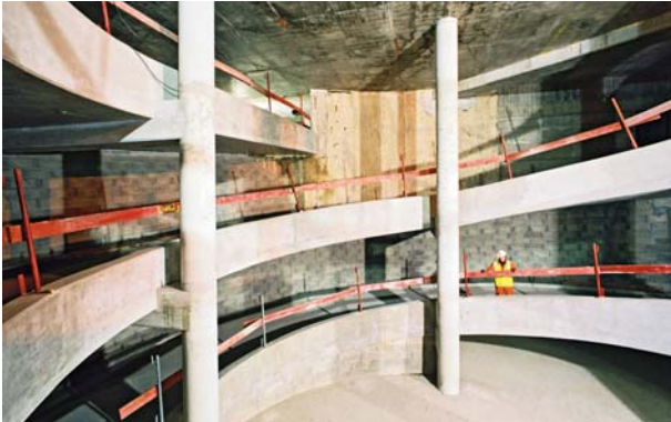
FRANCE - Boulogne-Billancourt Seguin car park
