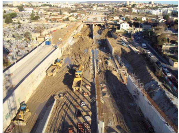
FRANCE - Marseille La Parette cut and cover
