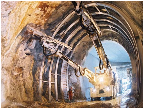
MONACO T33 tunnel
