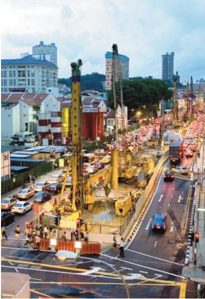
SINGAPORE - Downtown Line Cross Street Station & Tunnels (C908)
