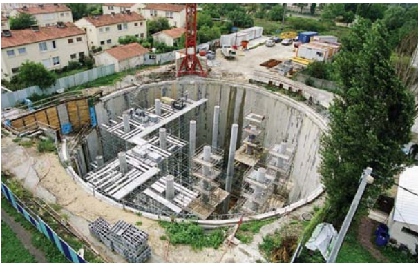
FRANCE - Bordeaux - Floirac Storage tank Alfred Giret
