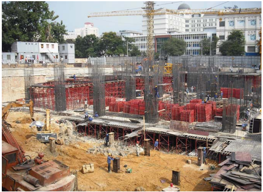
Earth moving in the excavation and structural works
