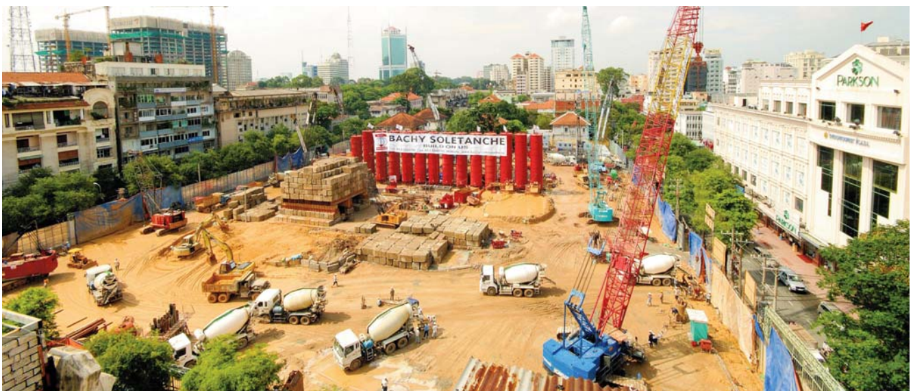
Site overview (load test in the center)
