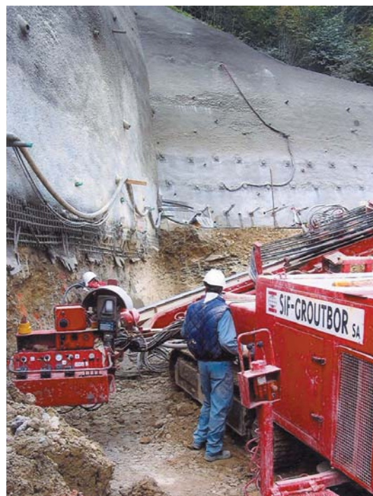
Carrying out the drilling (Casagrande C6 drilling machine)
