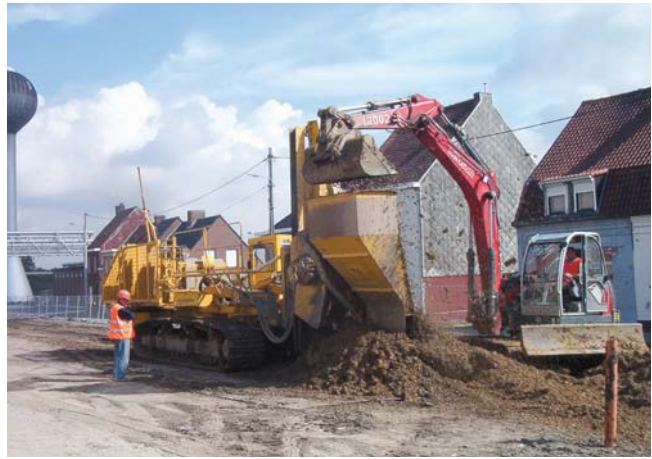
Installation of the drains
