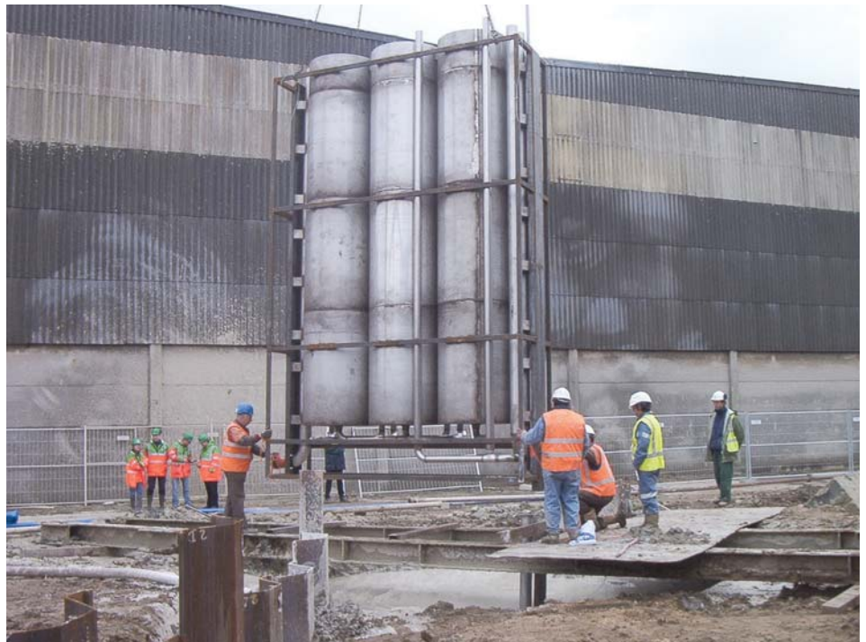
Placing of the filter gate
