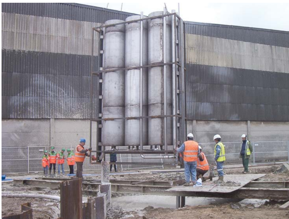
Placing of the filter gate
